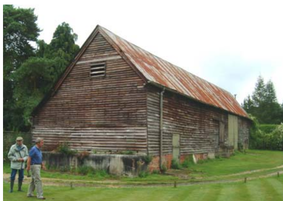
A timber framed barn formerly thatched and part of an agricultural group at Eastcourt Farm now attached to Weldermill Cottage.
