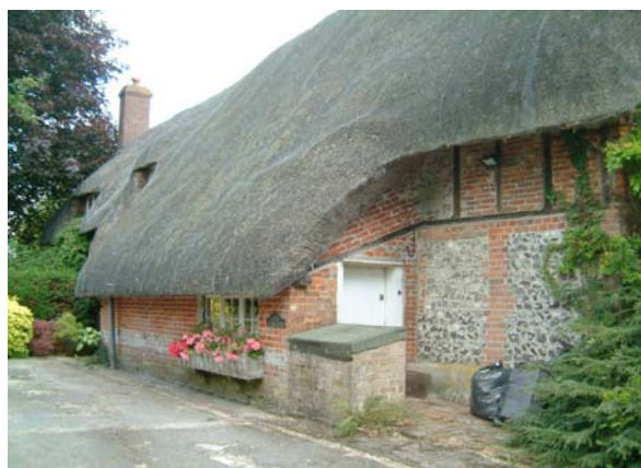
Yew Tree Cottage. Thatched roof and flint wall
