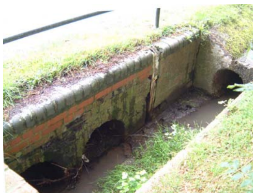
The culvert for stormwater outside Bridge Cottage. Ham is at a low level in the surrounding countryside and flooding can occur at this point in the village. Regular maintenance of the watercourses is particularly important.
