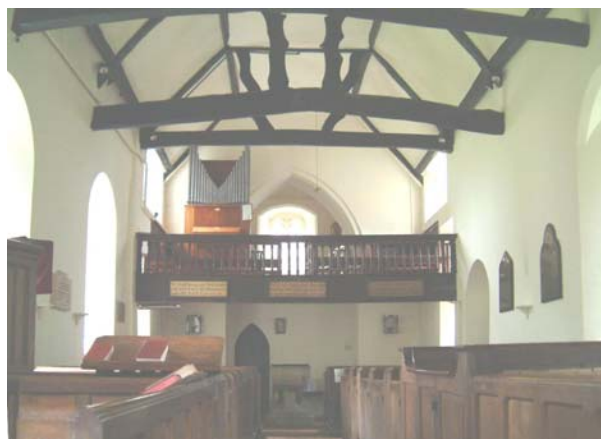
All Saints Church. The nave roof structure, the 18 th century gallery, pulpit, font and the box pews
