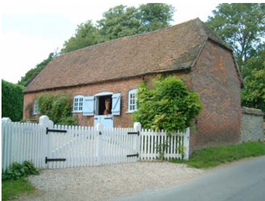
Plain clay tiles cover a half hipped roof over an early 19 th century stable
